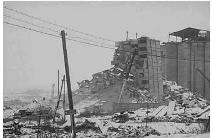
Fig. 1.2-7 Five-story building in Spitak, Armenia, destroyed during the December 7, 1988, earthquake. The building was made from precast concrete frames that were inadequately connected. The failure of such buildings contributed greatly to the loss of 25,000 lives. (Courtesy of the US Geological Survey.)
